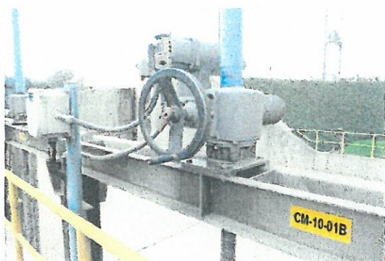
COMPUERTAS MOTORIZADAS (BYPASS) CM-10-01 B
